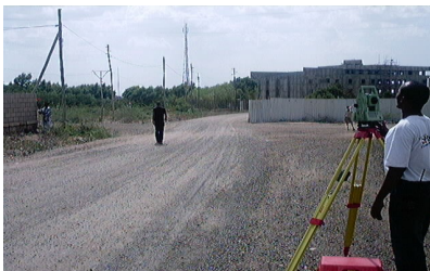
Surveying work in the expansion areas of the city
